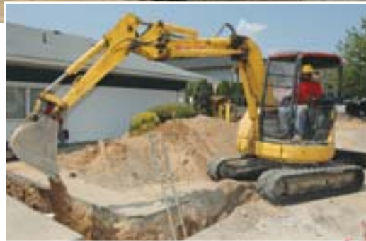
Operator Ramon Dominguez uses the company's Komatsu PC58UU compact excavator to backfill 160 feet of 12-inch water main at a customer's jobsite in Upper Saddle River, N.J.
